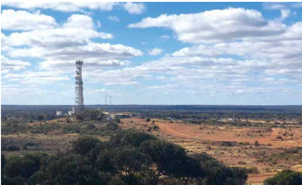
Telecommunications tower at Kalgoorlie, WA
